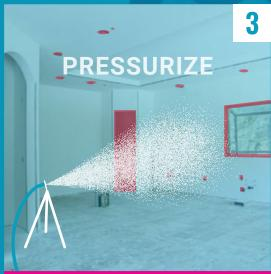
Use the computer-controlled atomization system to pressurize the space and spray. Sealant particles automatically seek out and find air gaps and holes up to ½" in size
