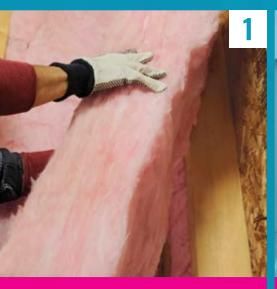
Install PINK® Fiberglas® Batt or Blown-in Insulation to local code requirements. Complete drywall installation and first mud application.\*
